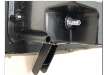
Make sure the back box sits straight and flush in the wall recess.
